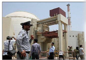
An Iranian security man stands next to journalists outside the reactor building at the Iranian-built Bushehr nuclear power plant in southern Iran on August 21, 2010. The Stuxnet computer worm has infected
